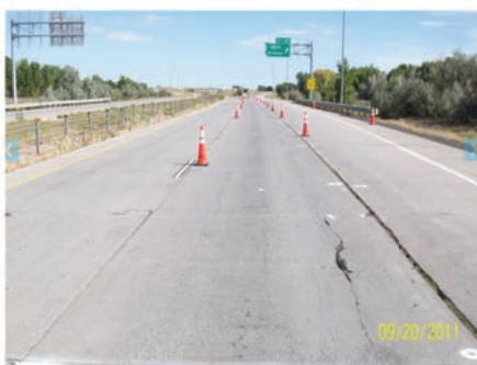
Figure 26. Longitudinal cracking near the shoulder in Colorado-0218 section (September 20, 2011).
