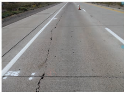
Figure 21. Longitudinal cracking near the shoulder in Arizona-0213 section (February 16, 2011).
